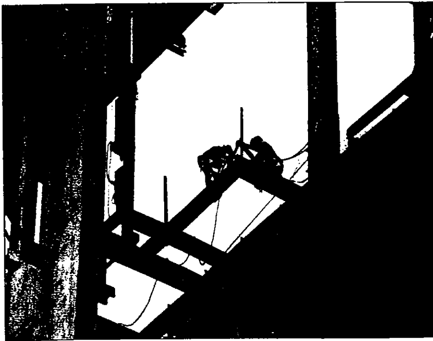
Ironworkers are erecting over 17,000 tons of steel on the structure. (Photo by Tom Hale)
